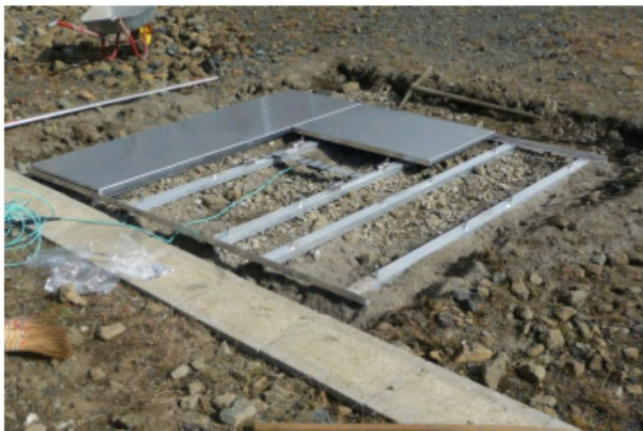
Figure 3: Preparation measuring site
